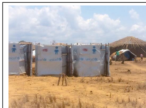
Latrines in IDP site, Metuge, October 2020.
